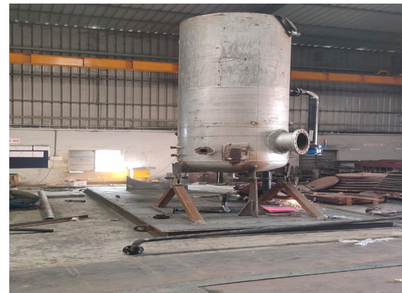
Separator Skid Fabrication works
