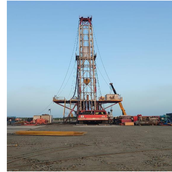
Rig Up at Elao drill site Drilling underway
